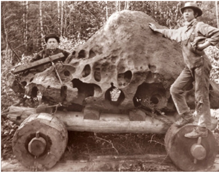
1903 - After digging around the 16 ton mass, Hughes and his teenage son , Elias (standing on wheel), jacked and levered the meteorite out of the hole onto a primitive flat-bed cart that they built entirely out of logs.
